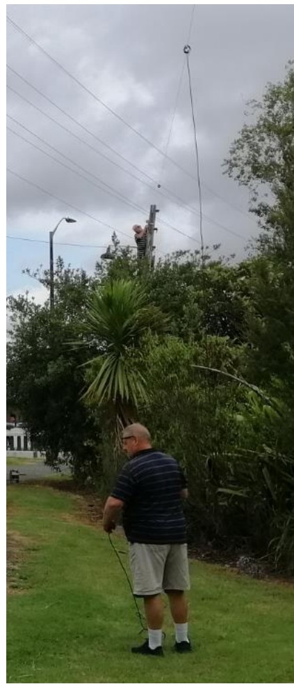
Tony ZL1TLC controlling the Coaxial cable as the Antenna was raised
